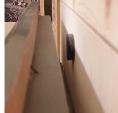
Too large distance:
